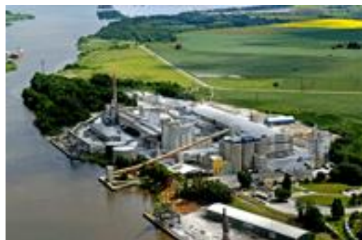
Figure 1 Nordkalk industrial area, located in Köping (Sweden), hosts Cortus' pilot plant
