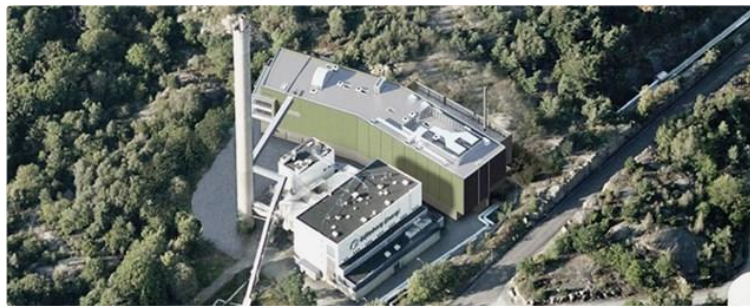
Figure 11 GoBiGas facility in Göteborg.
